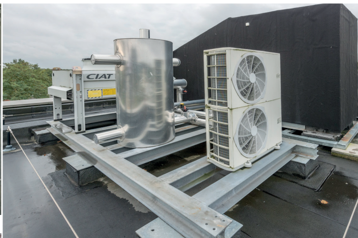
Machine froid + free cooling
